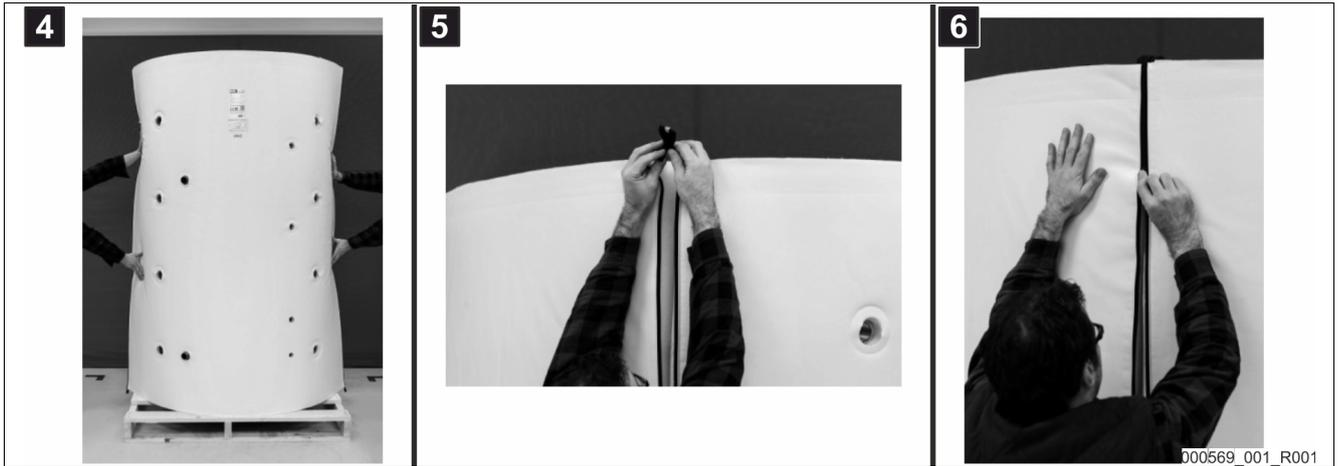
1. Distribute the thermal insulation uniformly over the entire circumference of the tank [4].
