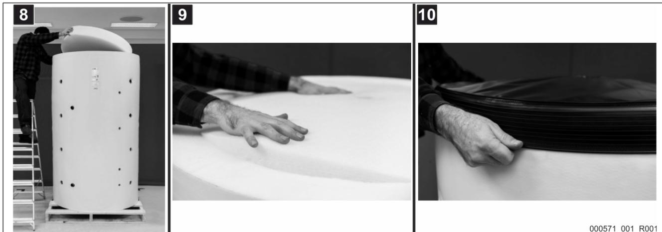
4. Position the top thermal insulation disc [8], [9].
